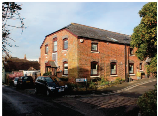
The Maltings on Drift Road, part of the former brewery
