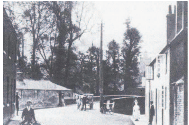
Wallington Bridge and adjacent cottages in the early 20 th century
