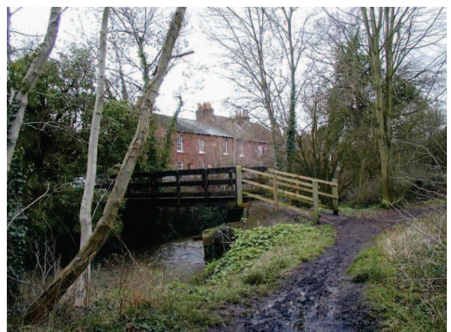
North Wallington viewed from the footpath to the water meadow
