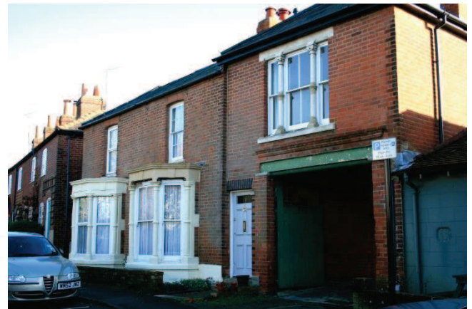
45 North Wallington –Formerly the Brewery Manager's House
